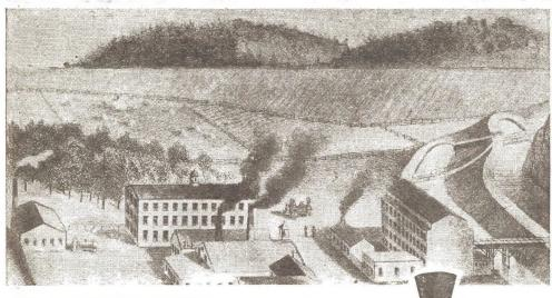
FIRM of Rogers, Ketchum & Grosvenor occupied old "Jefferson Works." Two raceways providing water power are at the right with the high embankment of the Morris Canal behind them
