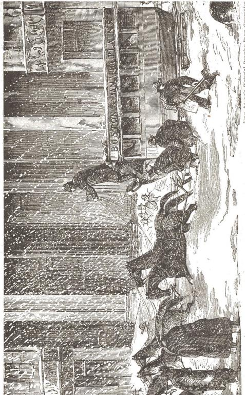
WINTER STREET, BOSTON, IN 1857. When heavy snow cove red the tracks, some cars were converted into sleights, their wheels From Builou's Pictorial Drawing-Room Companion being removed and bodies mounted on runners
